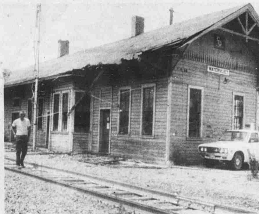
Swaying carriers damage depot roof.
