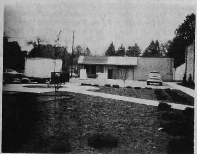
ALMOST COMPLETED...is the new Watervliet Public Library, the inside and outside work is nearly done, flowers will soon be planted in the front park and workers figure to be done by July 1. (Photo by Anne Bayer)
